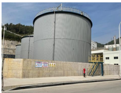
液硫罐区围堰4162m 3
