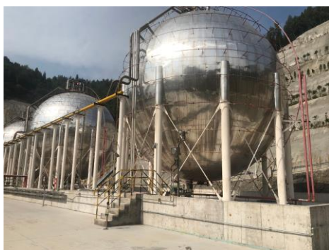
氨罐区围堰3000m 3
